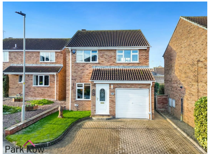
To the front of the property there is a block paved driveway with space for parking, access into the garage, a paved pathway which leads to the rear garden, a perimeter brick built dwarf wall to the left hand side, an outdoor light and the rest is mainly lawn.
